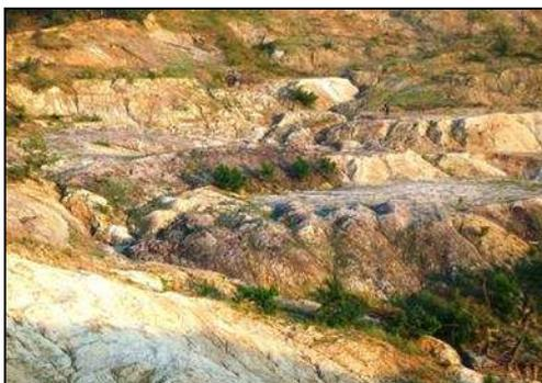
**Figure 4.** Steep embankment affected by erosion in the Budoi quarry
