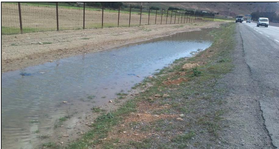
Figure 4. The stagnation of surface water on the edges of a poorly constructed roads
