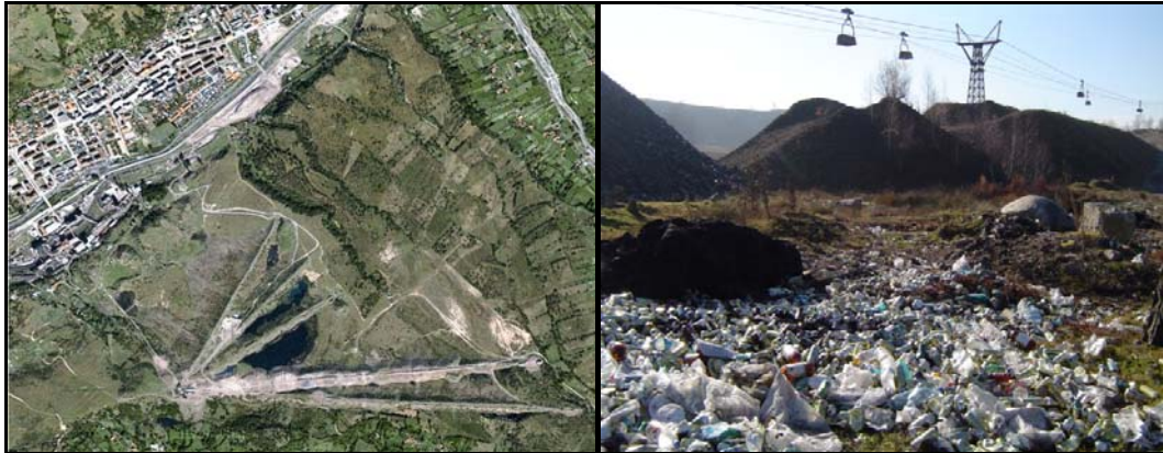
Figure 2. Structural and functional modification of geomorphologic environment in the area of Petrila town (Source: www.google.com/earth )
