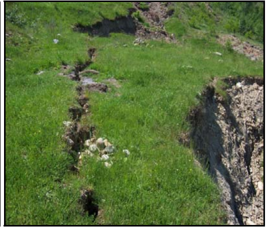
Figure 5. Collapse at the Defor coal pit
