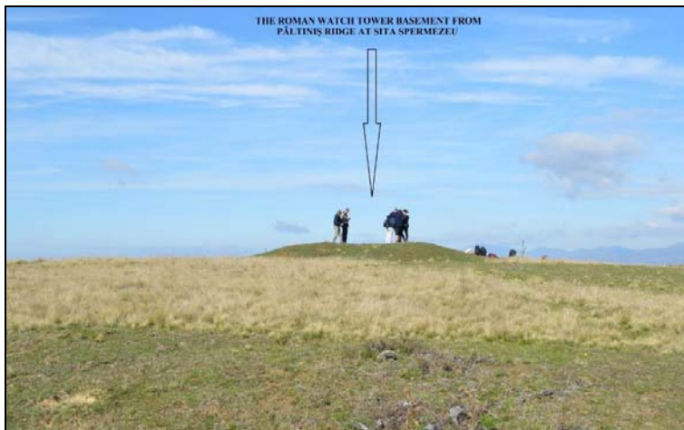
Figure 10. The substructure of the Roman tower on the Pălteniș Crest, at Sita Spermezeului
