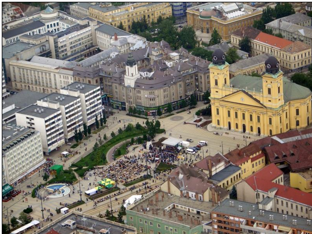
Figure 1. Renewed city centre with the Reformed Great Church 1
